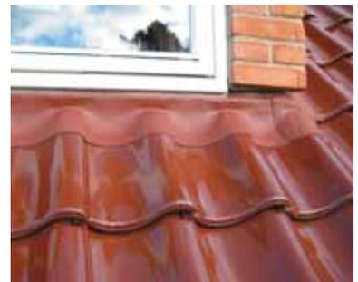
**Top:** *PERFORM flexible* roof flashing can be joined with all kinds of materials by using a silicon Adhesive. On the picture above this is used both for sealing at the exhaust and to assemble *PERFORM flexible* roof flashing in the corners of the roof covering sheet.
