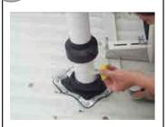
Slide the Support Cap down the pvc pipe. This will add extra support to the overall construction of the top hat roof kit. Glue in place using PVC solvent cement. 8
