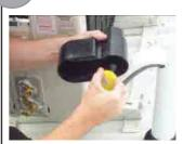
Apply pvc solvent cement to inside neck of Top Hat cap and to pvc pipe.
