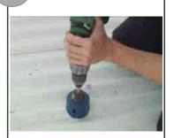
Cut hole in the roof sheet using hole saw or tin snips. Make sure the roof is free from any metal debris when complete.
