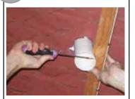
Secure pvc pipe within ceiling space to purlin rafter or truss. This will ensure the pvc will not drop or move over time.
