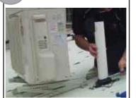
Align pvc pipe for connection of services to machinery, making sure the service entry point is facing the unit.
