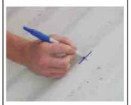
Mark the cut out in the roof sheet away from the screw line. Make sure the centre of the cut out is on the raised section of the roof profile and does not sit on over lap of roof sheets.
