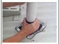
Trim the cone of the Dektite to suit pipe size using sharp tin snips. Slide down pipe using water as a lubricant. Apply sealant by turning back flexible flange. Press base to the roof profile by hand then fix to the roof using screws provided.
